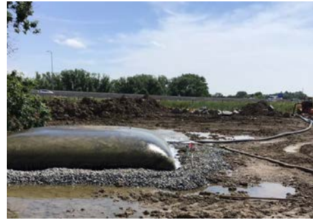
Pumped water filter bags remove coarse sediment from water pumped from site locations like foundations, vaults, and trenches.
