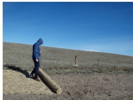
Installation of slope stabilizing erosion control blankets.
