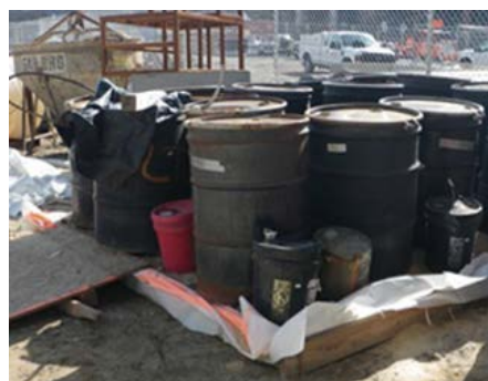
Secondary containment used to capture any spills.
