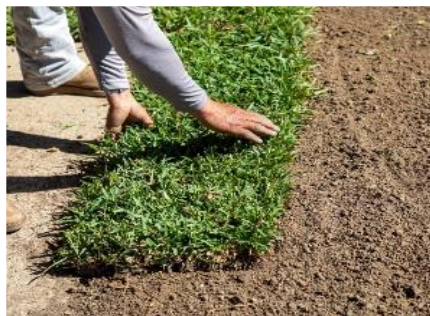
Sod can be used to quickly stabilize soil and reduce erosion.
