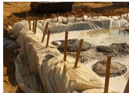
When washout basins are full, cover the basin and direct future washout wastes to a new one.
