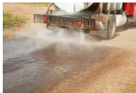
A water tanker truck wetting high traffic areas for dust suppression.
