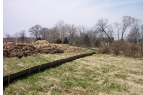
Proper silt fence installation at the perimeter of a construction site.
