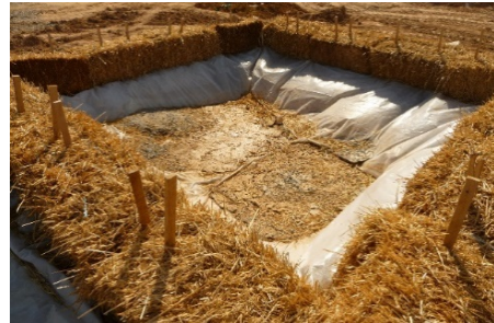
Concrete washouts can be fabricated from straw bales, plastic sheeting, and wooden stakes.
