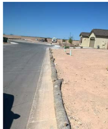
Sediment filter logs at the edge of a residential construction site reduce the sediment carried onto the street by stormwater.
