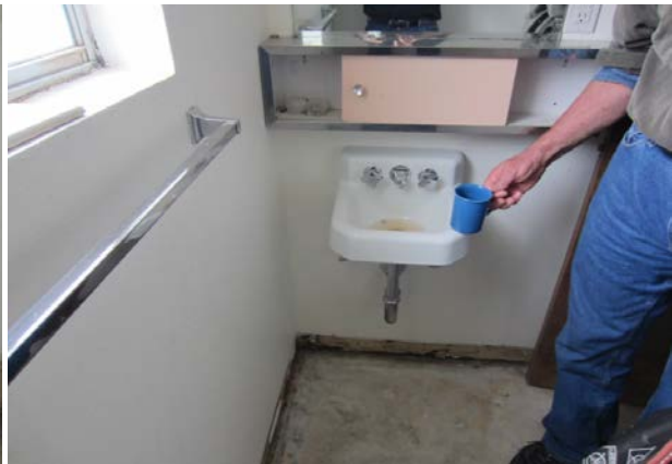
Figure 8 – Main House (unfinished RR)
