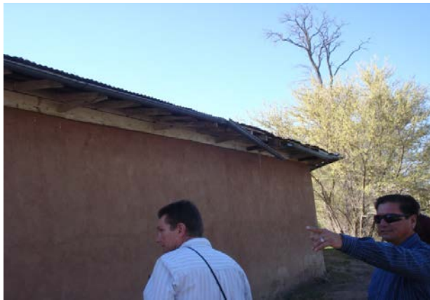
Figure 7 – Adobe Storage Buildings
