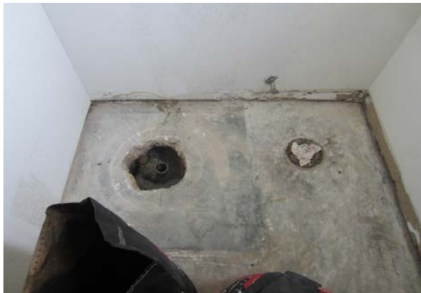
Figure 7 – Main House (unfinished RR)
