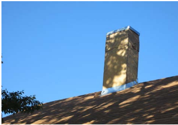
Figure 1 - Main Home Chimney
