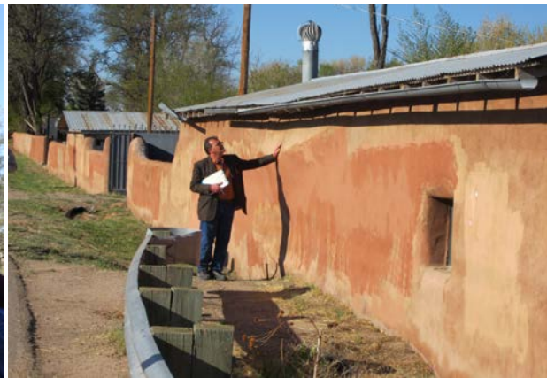
Figure 8 – Adobe Storage Building & Fence
