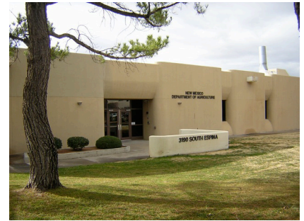
Existing building exterior
