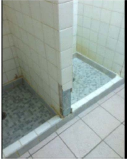
1) FOOTBALL COACH'S LOCKER ROOM (REPAIRED NOW)
