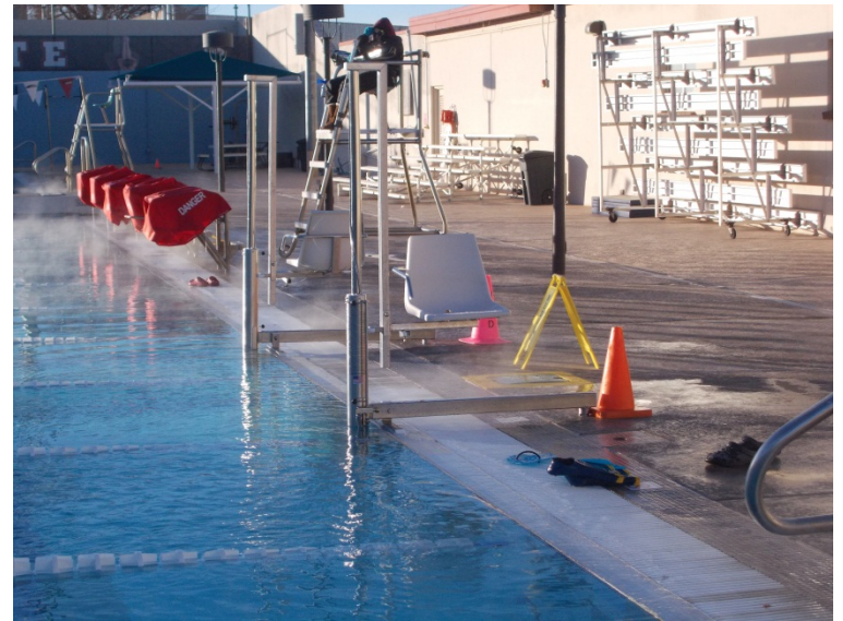
Aquatic Center ADA Pool Lift
