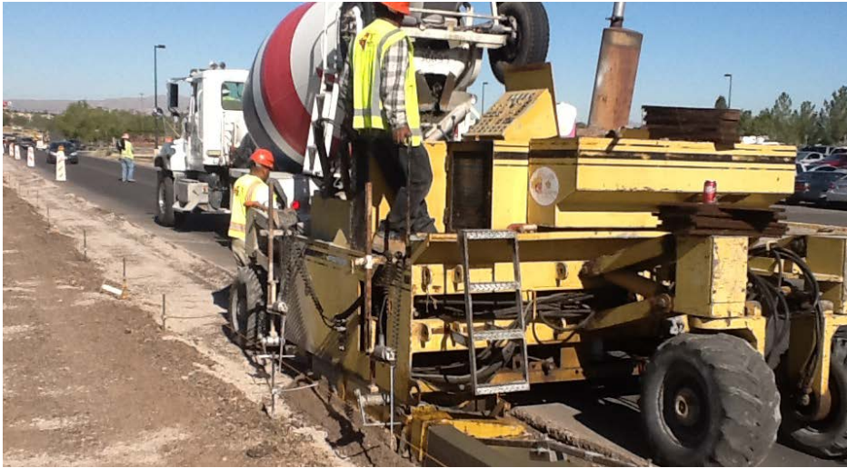
Sam Steel Curb and Gutter Replacement
